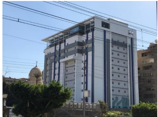
Cairo Specialized Hospital Post-Renovation
