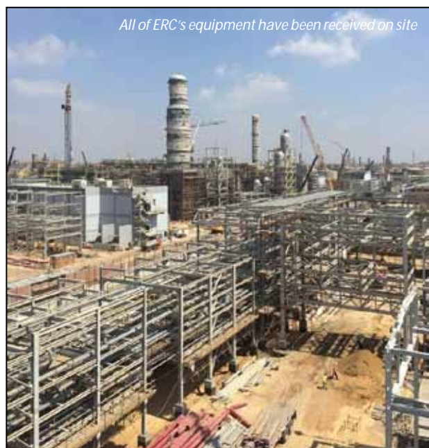
ERC's construction site
